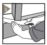
Lay a loose board upside down as a proper height guide against the door jamb. Cut the bottom of the frame off, leaving the required expansion gap allowance.
